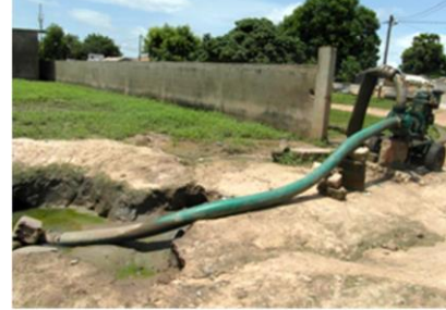
Photo 5: Water pumping device in the flooded area of Diamaguène Centre - School 5
