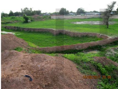
Photo 4: Rainwater retention and drainage basins and concrete protection dam against runoff.
