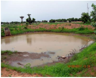
Photo 3: Retention basins and overflow of pumped water from flooded areas
